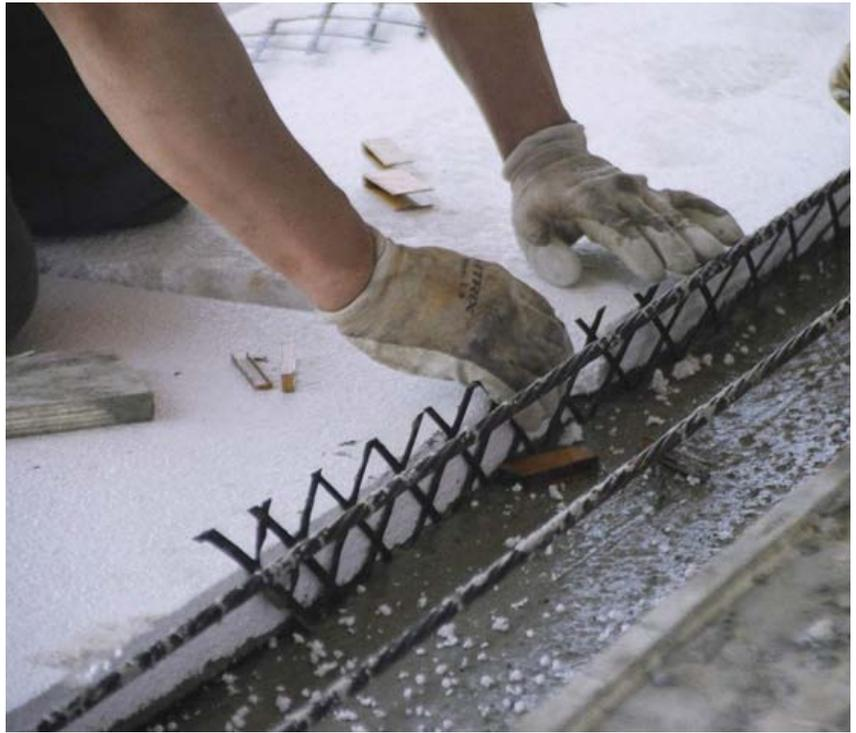
**Right:** Carbon fiber grid connectors and EPS insulation
