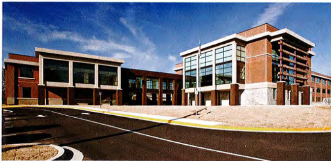
The precast panels on Tucker High School incorporated integral architectural finishes, including thin-set brick and exposed concrete to emulate limestone
