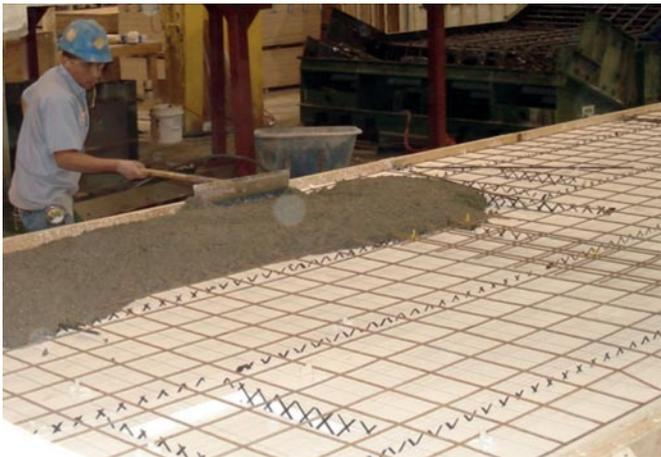
Fig. 2: Casting the Inner Wythe Concrete in a Sandwich Wall Panel using CFRP Wythe Connections
