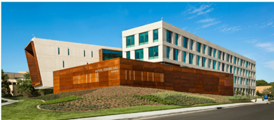
Capitol Federal Hall, University of Kansas School of Business in Lawrence, Kansas, USA, uses CarbonCast High Performance Insulated Wall Panels shows how insulated panels can deliver the same aesthetic as conventional architectural cladding while offering energy savings. (Precaster: Enterprise Precast.) © Jacia Phillips.
