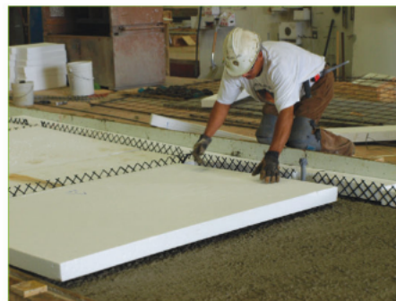
Expanded polystyrene insulation is placed atop the poured outer wythe with the carbon fiber grid embedded. The inside concrete wythe will be poured atop the insulation; the grid connects the two wythes through the insulation.
