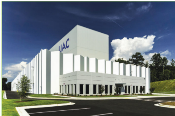
The Universal Alloy Light Press Plant in Ball Ground, Georgia, USA, features load-bearing CarbonCast High Performance Insulated Wall Panels painted to create a 3-D illusion. The carbon fiber grid wythe connectors contribute to the building's R-11 performance. (Precaster: Metromont)
